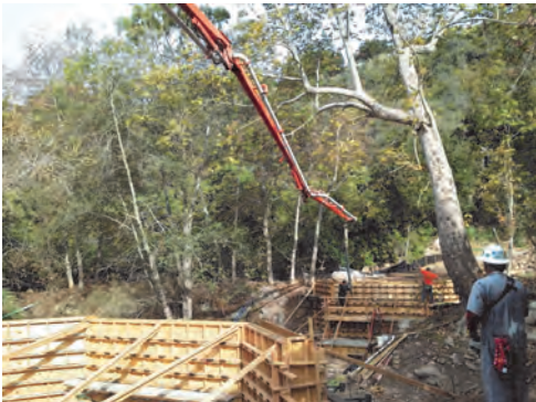
POURING OF THE CONCRETE ABUTMENTS FOR THE BRIDGE
