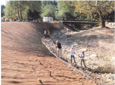
THE TOP LEFT PHOTO SHOWS CROSSING T-7 JUST AS DEMOLITION OF THE CONCRETE BEGAN. THE MIDDLE PHOTO SHOW THE NEW BRIDGE THAT WAS INSTALLED NEAR THE LOCATION OF THE FORMER CROSSING, LOOKING UPSTREAM. THE RIGHT PHOTO SHOWS THE CALIFORNIA CONSERVATION CORPS WORKING TO INSTALL A WILLOW MATTRESS UPSTREAM OF THE NEW BRIDGE, AN ADDITIONAL BIOTECHNICAL BANK STABILIZATION METHOD THAT WAS EMPLOYED BY THE PROJECT.
