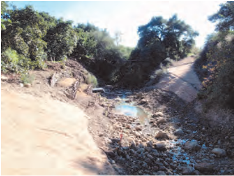
THE TOP LEFT PHOTO SHOWS CROSSING T-6 BEFORE CONSTRUCTION FACING DOWNSTREAM. ALL THE CONCRETE AND THE ROCK AND METAL REVETMENT WAS REMOVED AS PART OF THE PROJECT. THE MIDDLE PHOTO SHOW THE REGRADED STREAM CHANNEL AFTER CONSTRUCTION AND INSTALLATION OF EROSION CONTROL MATERIAL. THE RIGHT PHOTO SHOWS THE WILLOW WATTLE FENCE THAT WAS INSTALLED AT THE SITE AS A BIOTECHNICAL BANK STABILIZATION ALTERNATIVE TO REVETMENT.
