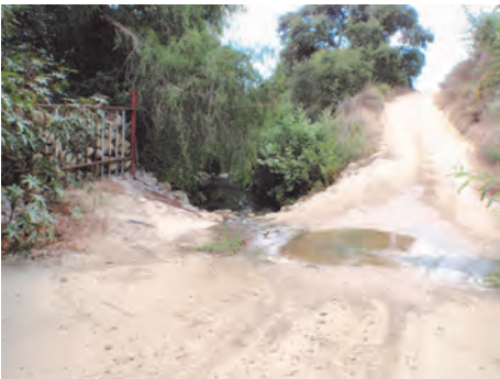
THE TOP LEFT PHOTO SHOWS CROSSING T-6 BEFORE CONSTRUCTION FACING DOWNSTREAM. ALL THE CONCRETE AND THE ROCK AND METAL REVETMENT WAS REMOVED AS PART OF THE PROJECT. THE MIDDLE PHOTO SHOW THE REGRADED STREAM CHANNEL AFTER CONSTRUCTION AND INSTALLATION OF EROSION CONTROL MATERIAL. THE RIGHT PHOTO SHOWS THE WILLOW WATTLE FENCE THAT WAS INSTALLED AT THE SITE AS A BIOTECHNICAL BANK STABILIZATION ALTERNATIVE TO REVETMENT.
