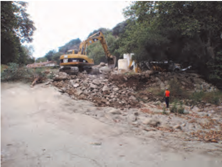
THE TOP LEFT PHOTO SHOWS CROSSING T-7 JUST AS DEMOLITION OF THE CONCRETE BEGAN. THE MIDDLE PHOTO SHOW THE NEW BRIDGE THAT WAS INSTALLED NEAR THE LOCATION OF THE FORMER CROSSING, LOOKING UPSTREAM. THE RIGHT PHOTO SHOWS THE CALIFORNIA CONSERVATION CORPS WORKING TO INSTALL A WILLOW MATTRESS UPSTREAM OF THE NEW BRIDGE, AN ADDITIONAL BIOTECHNICAL BANK STABILIZATION METHOD THAT WAS EMPLOYED BY THE PROJECT.
