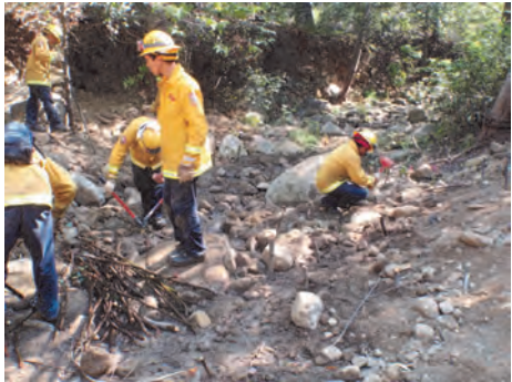
THE TOP LEFT PHOTO SHOWS CROSSING T-8 BEFORE CONSTRUCTION FACING UPSTREAM. THE MIDDLE PHOTO SHOW THE REGRADED STREAM CHANNEL AFTER CONSTRUCTION WAS COMPLETE. THE RIGHT PHOTO SHOWS THE CALIFORNIA CONSERVATION CORPS INSTALLING WILLOW STAKES AT THE SITE. THESE POLES BEGAN SPROUTING AFTER JUST A FEW WEEKS.
