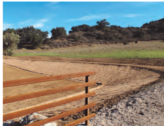
CCC MEMBERS INSTALLED EROSION CONTROL MATERIAL AND NATIVE SEED ON SLOPES IN THE PROJECT AREA
