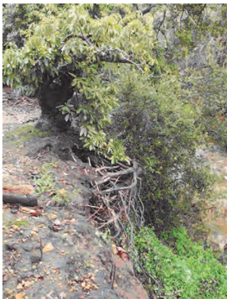
BEFORE PHOTO OF THE UPPER MOST SECTION OF THE PROJECT, SHOWING VERTICAL CREEK BANK AND UNSTABLE AVOCADO TREES AT THE TOP OF BANK.
