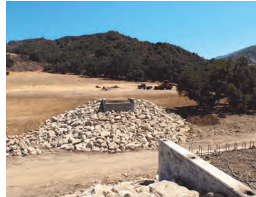
ABUTMENTS & ROCK SLOPE PROTECTION PRIOR TO BRIDGE INSTALLATION
