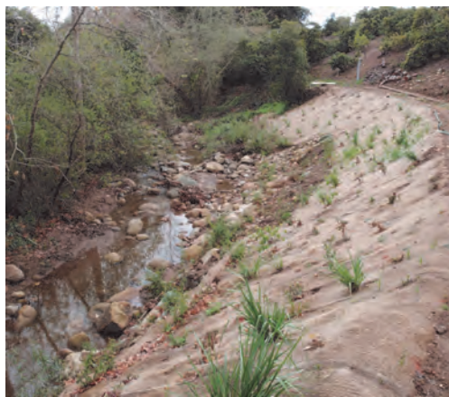
CATE BANK STABILIZATION PROJECT LOOKING DOWNSTREAM AT THE LOWER SECTION OF THE PROJECT. SHOWS A SIGNIFICANT AMOUNT OF GROWTH IN THE WILLOWS ALONG THE TOE OF THE SLOPE AS WELL AS FROM THE CONTAINER PLANTS PANTED THROUGHOUT THE SLOPE.
