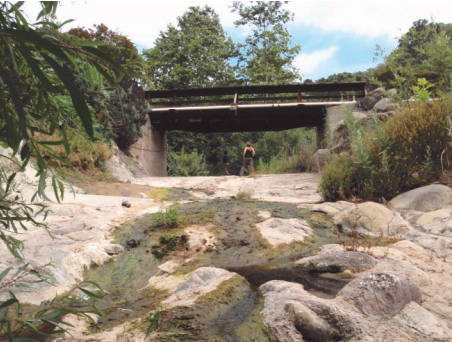
THE CURRENT PINKHAM CROSSING IS A COMPLETE BARRIER TO STEELHEAD PASSAGE.
